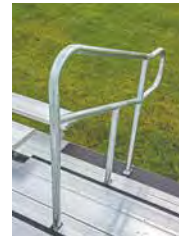
A Central Aisle & Sturdy Hand Rail are Good Safety Options.
